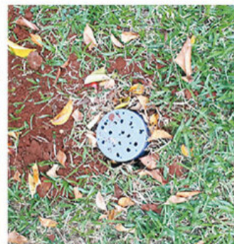
IEI employee digs hole for a biopore; a biopore in the ground
