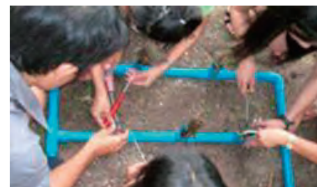
Assembling plastic pipes to create an artificial reef
