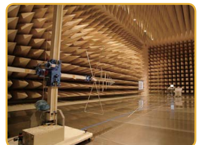
EMC testing facility
