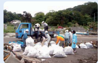
Debris removal (Kesenuma)
