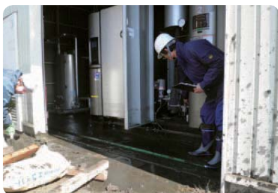
Restoration of inundated equipment
