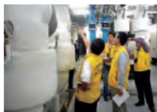
Photo 3. Taiwan Energy Patrol Team members on-site for energy assessment
