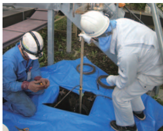
Maintenance of pumping equipment
