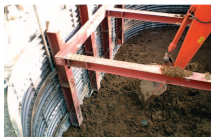
Soil removal work at the Suwa Minami Plant
