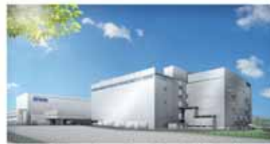
New factory planned at Hirooka Office (Japan) (Operations scheduled for FY2018)
